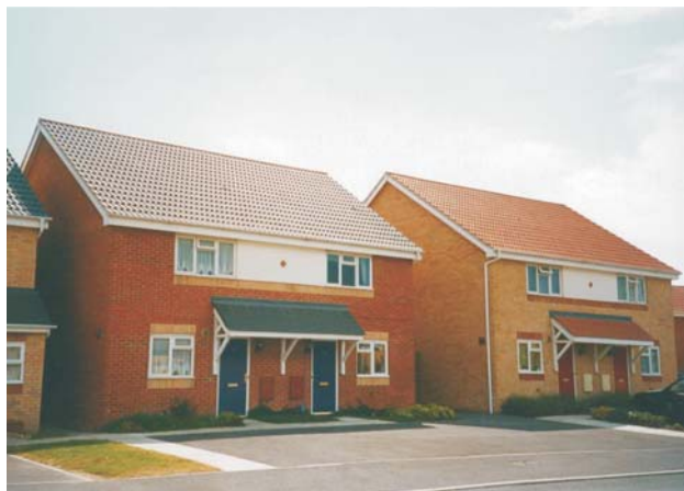
Figure 3.1: An example of housing built within the density range of 30 to 50 dwellings per hectare
