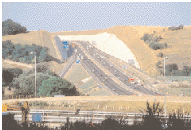
66. Road construction - Twyford Down
