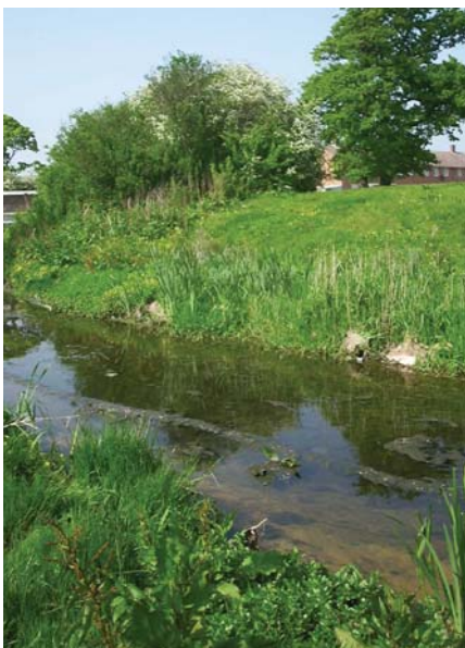
↑ Restored concrete lined channel on stretch of the Hermitage Stream.
