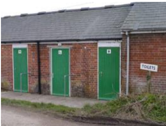
Existing toilets at Grange Farm complex
