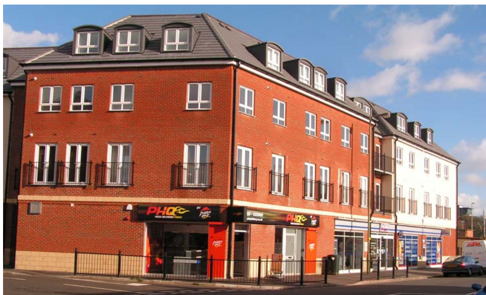
Figure 8.3: Co-op Foodstore, Forton Road
