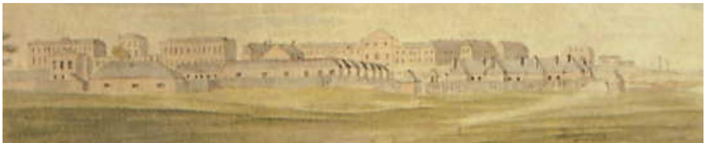
A view of Haslar Barracks from Monckton with Haslar Hospital in the distance. Detail from a watercolour by Captain John Durant, who served in the 2 nd West Riding Militia 1800-1814. This regiment was in garrison at Haslar in 1813 and 1814.
