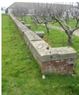
Plinth Wall for railing
