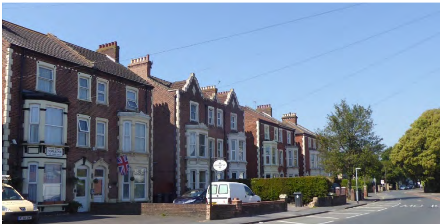
South side Bury Road (eastern end)
