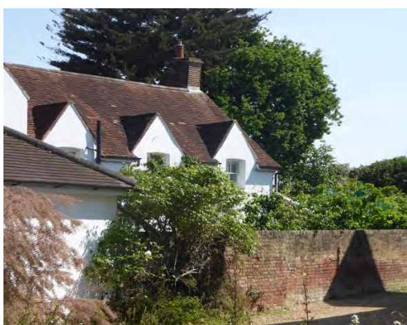
The older south range, to Bury Grange (now part of No.5)
