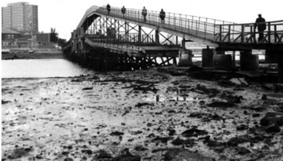
Haslar foot bridge, known as Pneumonia Bridge, about 1973
