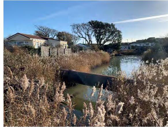
Remains of part of the Stokes Bay Lines Moat
