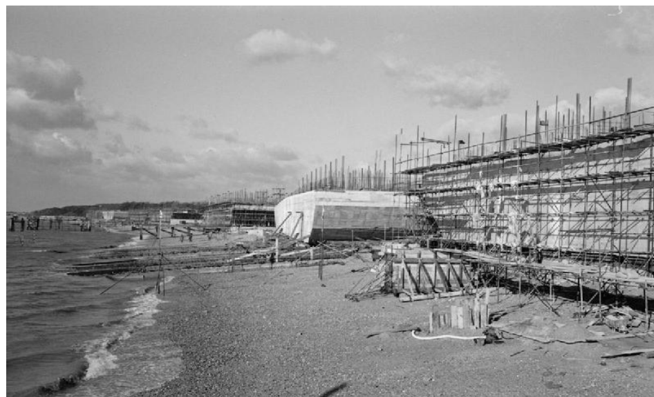
Phoenix caissons under construction at Stokes Bay (fortgilkicker.co.uk).
