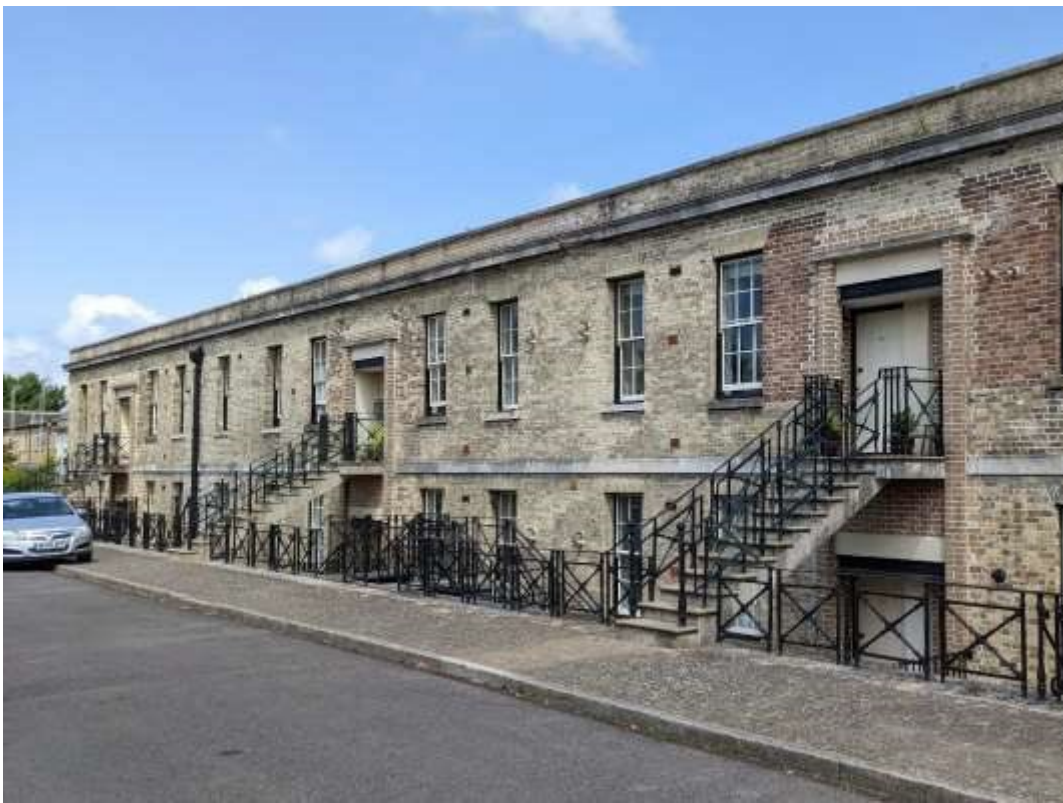
Figure 39 Grade II listed main barrack block
