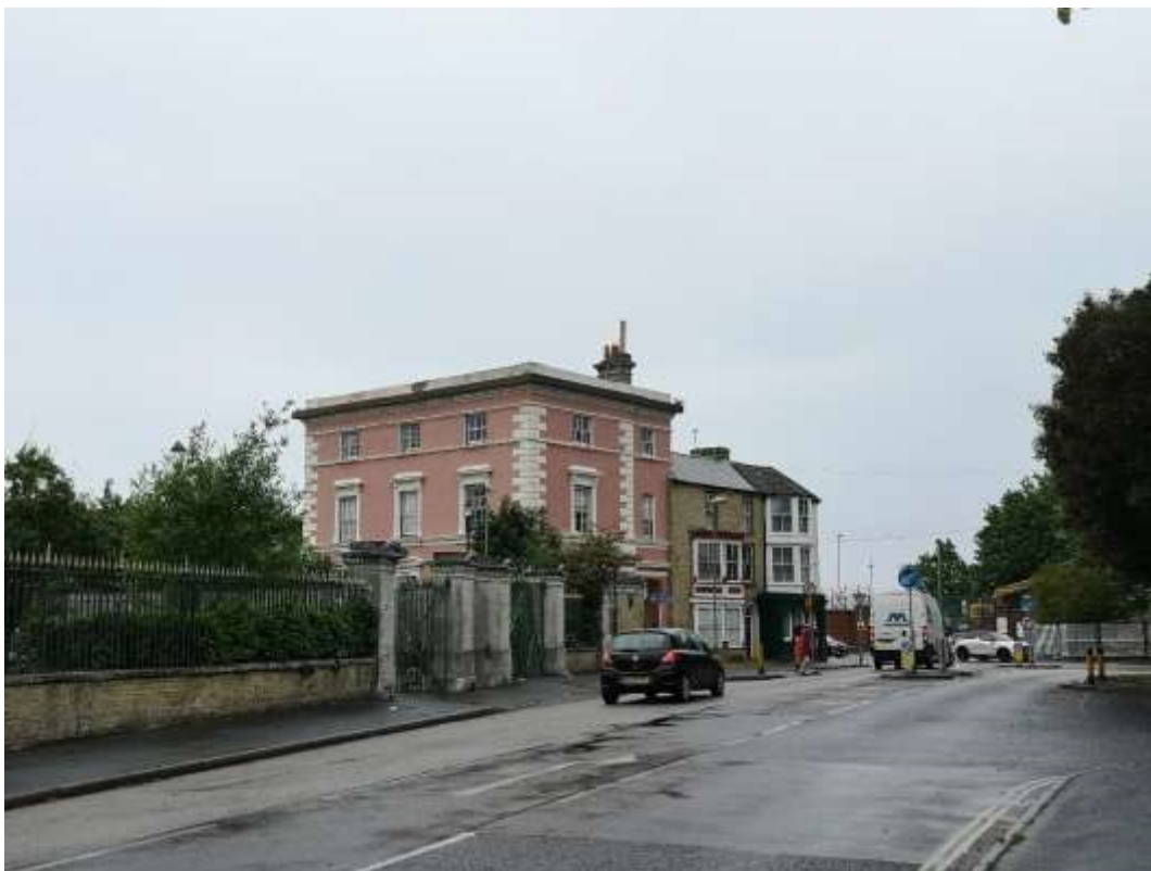
Figure 15 Railway Hotel, Railway Inn and Spring Cottage (each Grade II listed) on Spring Garden Lane
