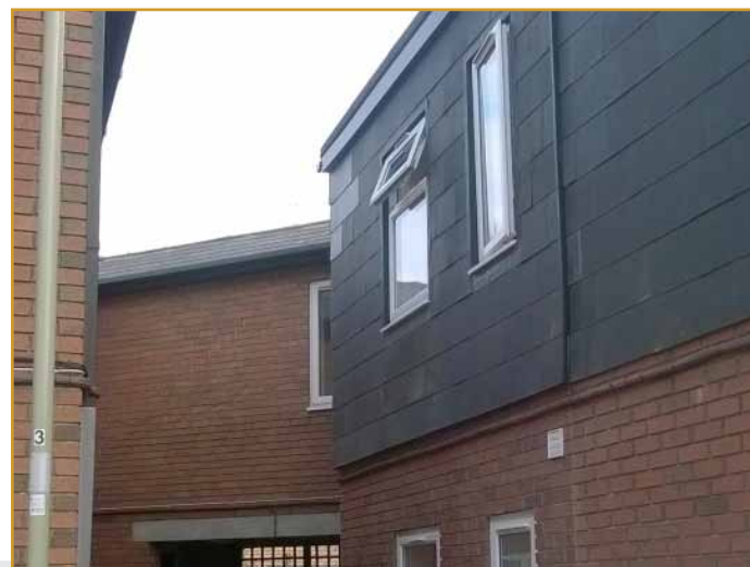
Gloucester House showing completed extension work
