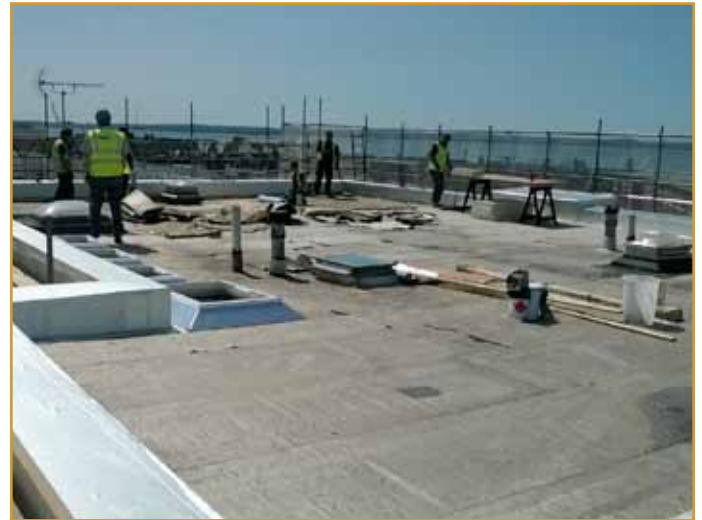
Hove Court roof undergoing repair
