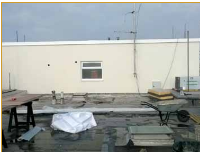
Finished wall insulation at Hove Court
