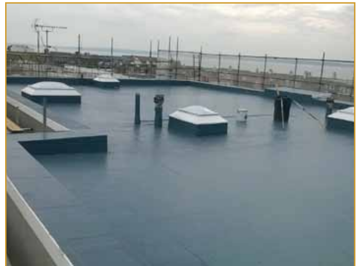
Completed roof at Hove Court
