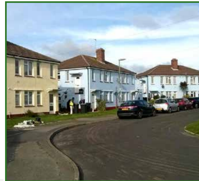
Completed works at Beryton Close
