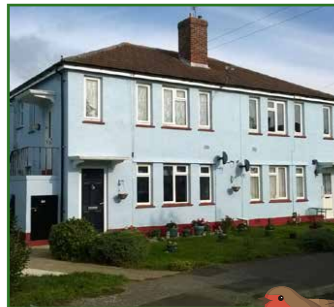
Completed works at Beryton Close
