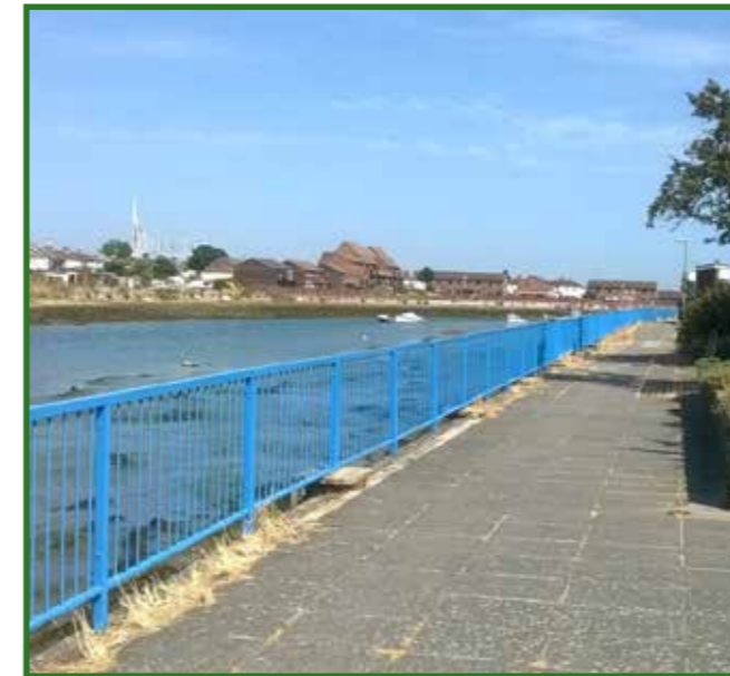
Completed railings that run alongside Dolphin Crescent
