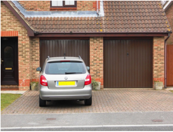
These garages are too narrow for a car and the driveway is too short to allow convenient access for cycle storage.
